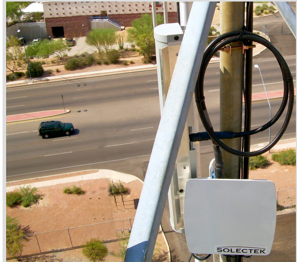
Above is an example of a SkyWay wireless mounted on a service pole.
