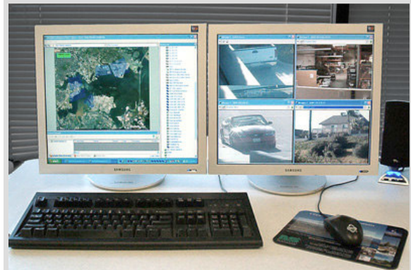
A typical video monitoring station is pictured above.
