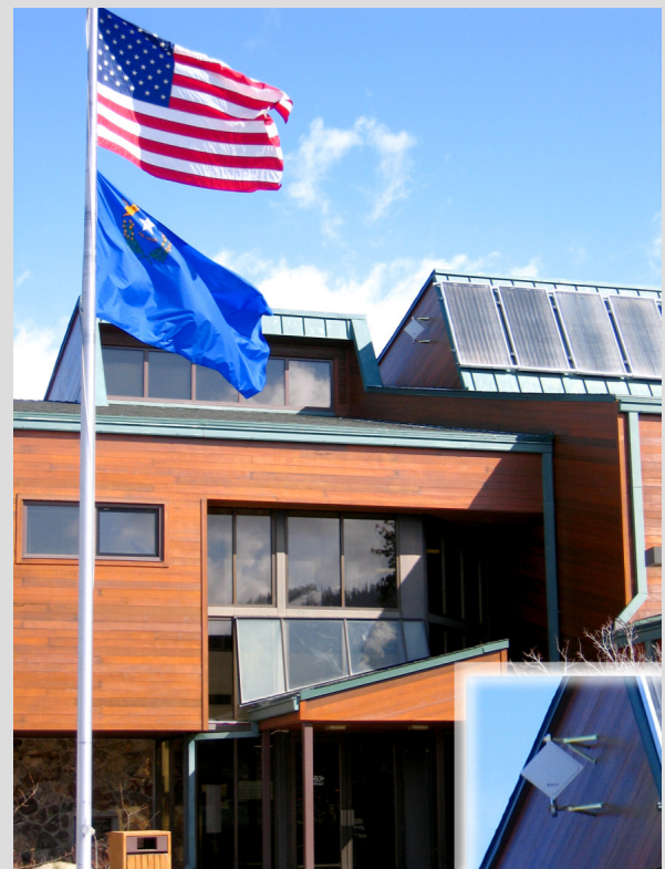
The Sheriff's office located in Stateline, NV. The radio unit is mounted near the top of the building (shown magnified in bottom right)
