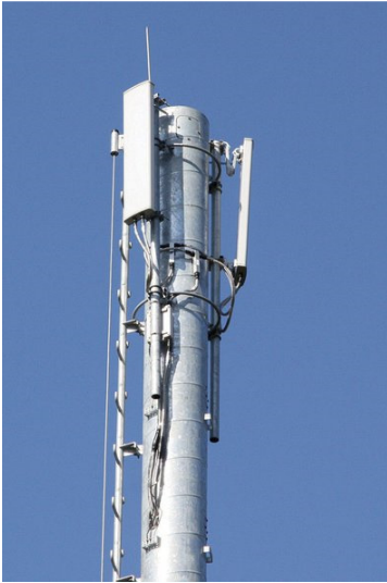
(Left) a simple three-sector base station on a mast, (Right) crowded tower site with PTP antennas
