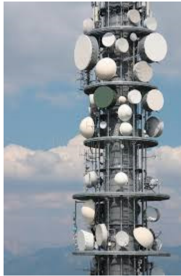
(Left) a simple three-sector base station on a mast, (Right) crowded tower site with PTP antennas
